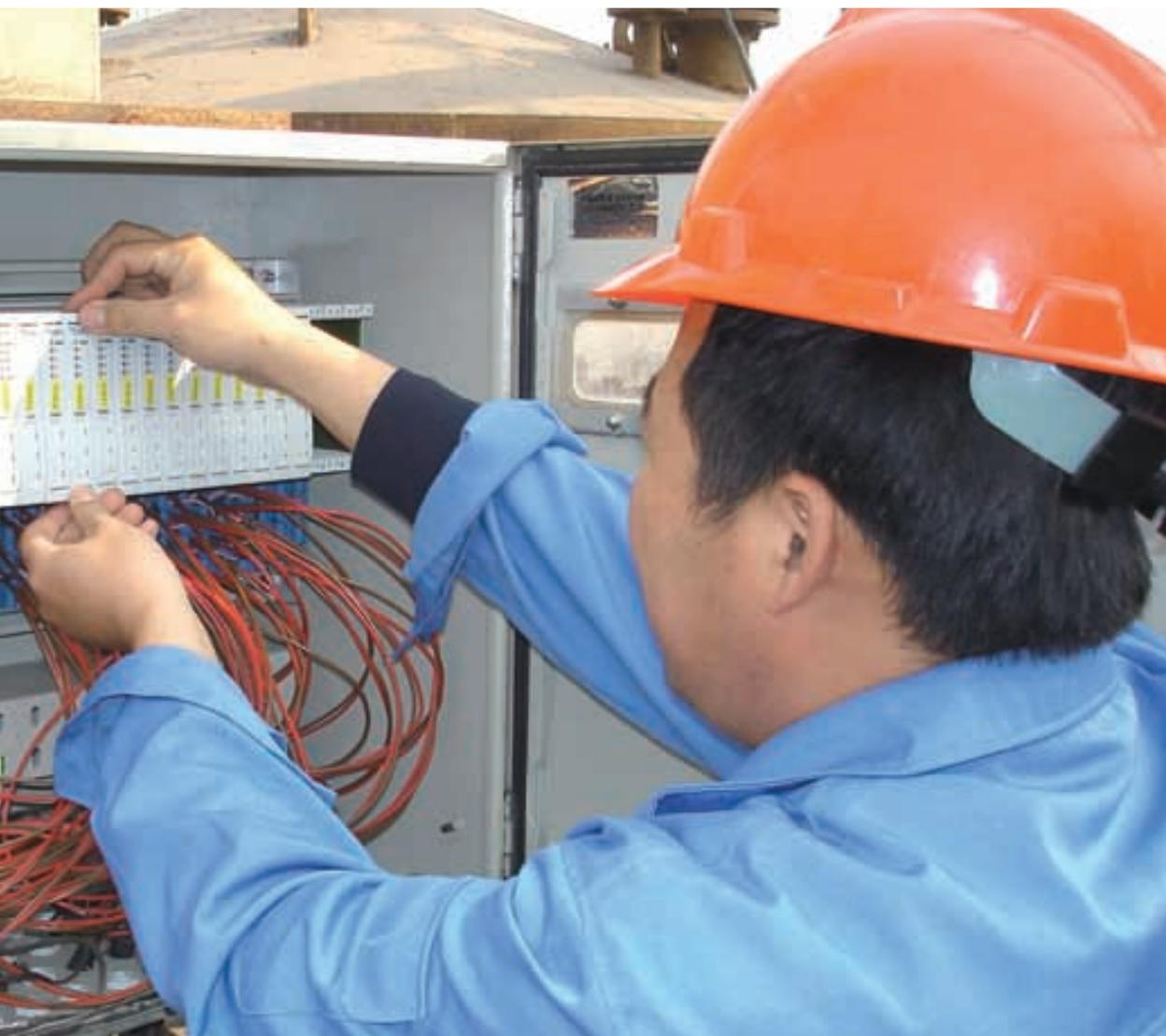
The advantage of the modular design of the excom station: The up to 16 I/O modules – including the power supply packs – can be replaced during continuous operation in Zone 1
