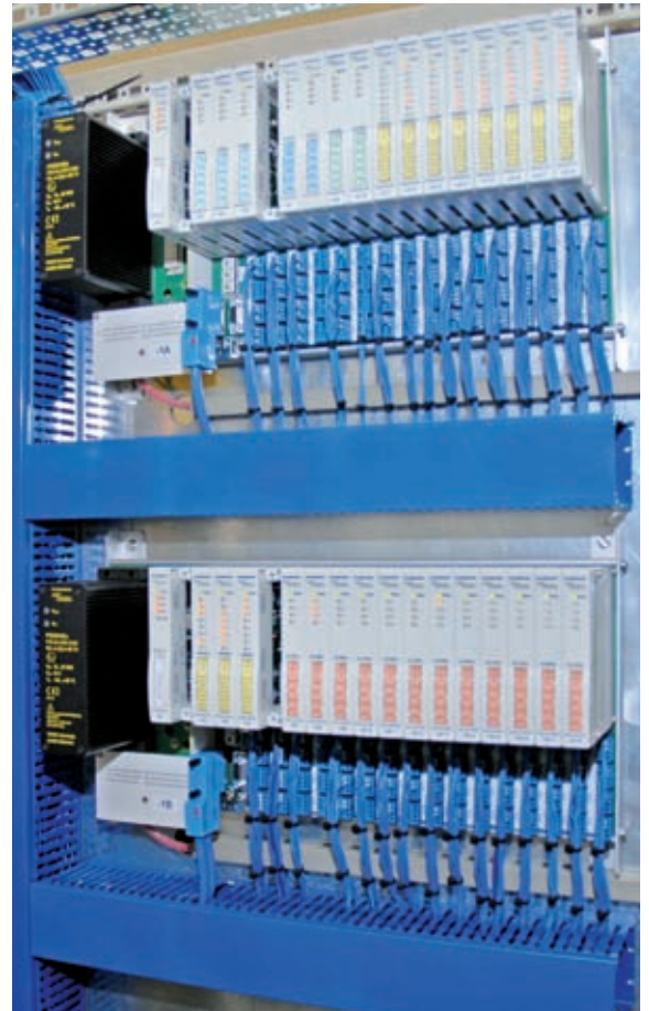
In only one weekend, EAB Automation installed the new excom systems into the 19" racks
